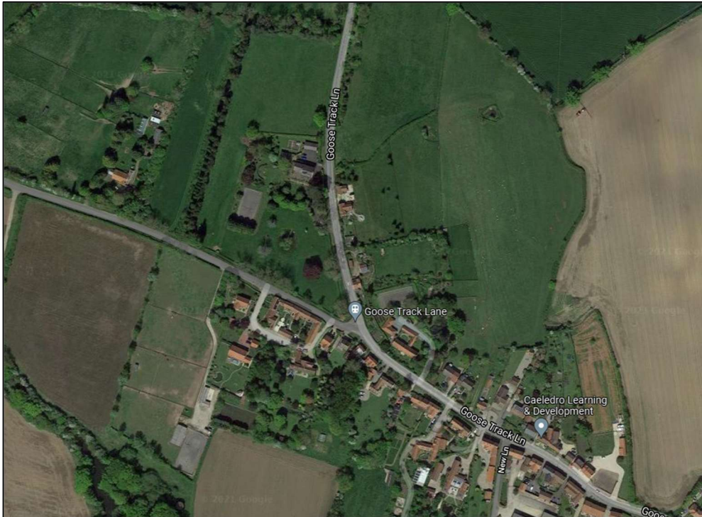
Image 3: Aerial View of Application Site
